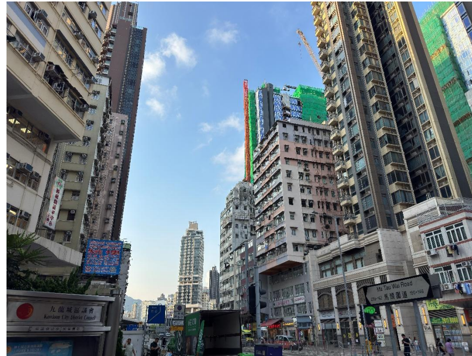
VP4 Junction between Ma Tau Wai Road and Bailey Street
